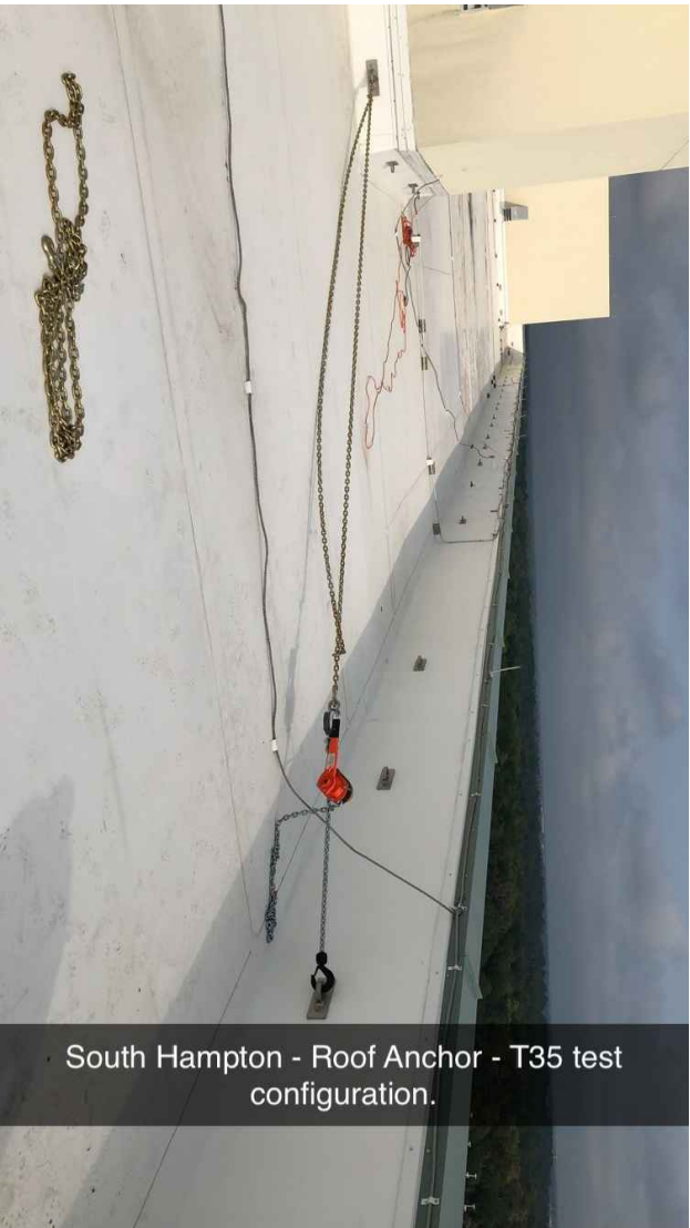
South Hampton - Roof Anchor #39 - post-test.
