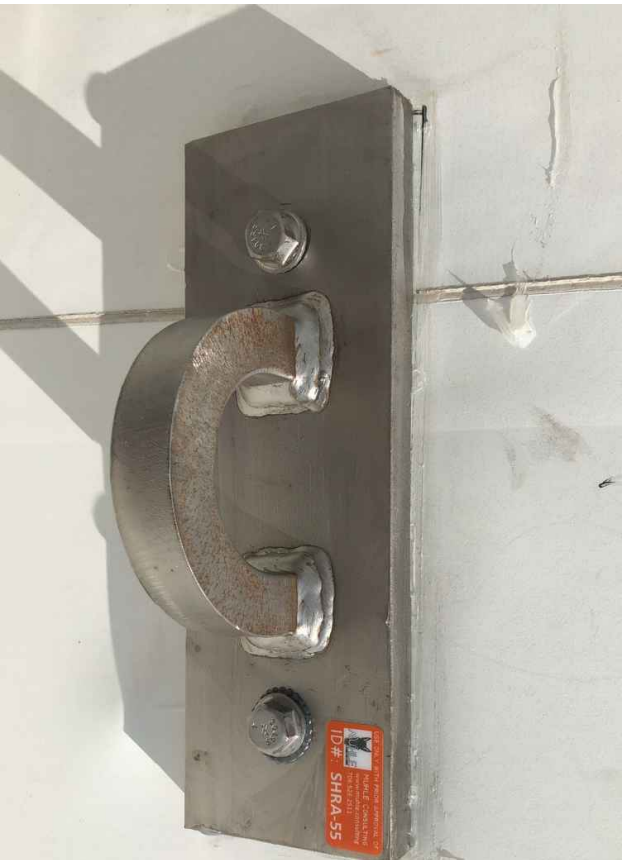
South Hampton - Roof Anchor #55 - post-test.
