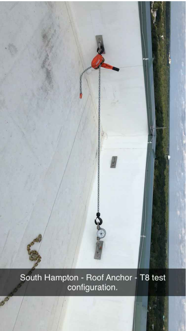
South Hampton - Roof Anchor #08 - post-test.
