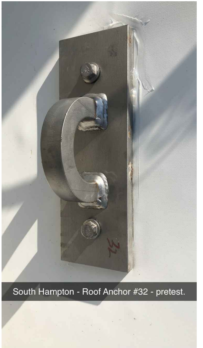
South Hampton - Roof Anchor - T32 test configuration.
