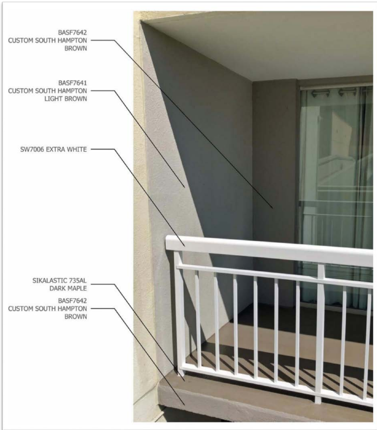
Figure #1 – Mock-Up at Unit #106
